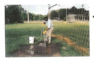
A hand pump and bucket can be used to remove water in areas where there are puddles. Once the bucket is full, dispose of the water <u>outside</u> the field of play. However, this will not make the field immediately playable, it will only accelerate drying of the affected area.
